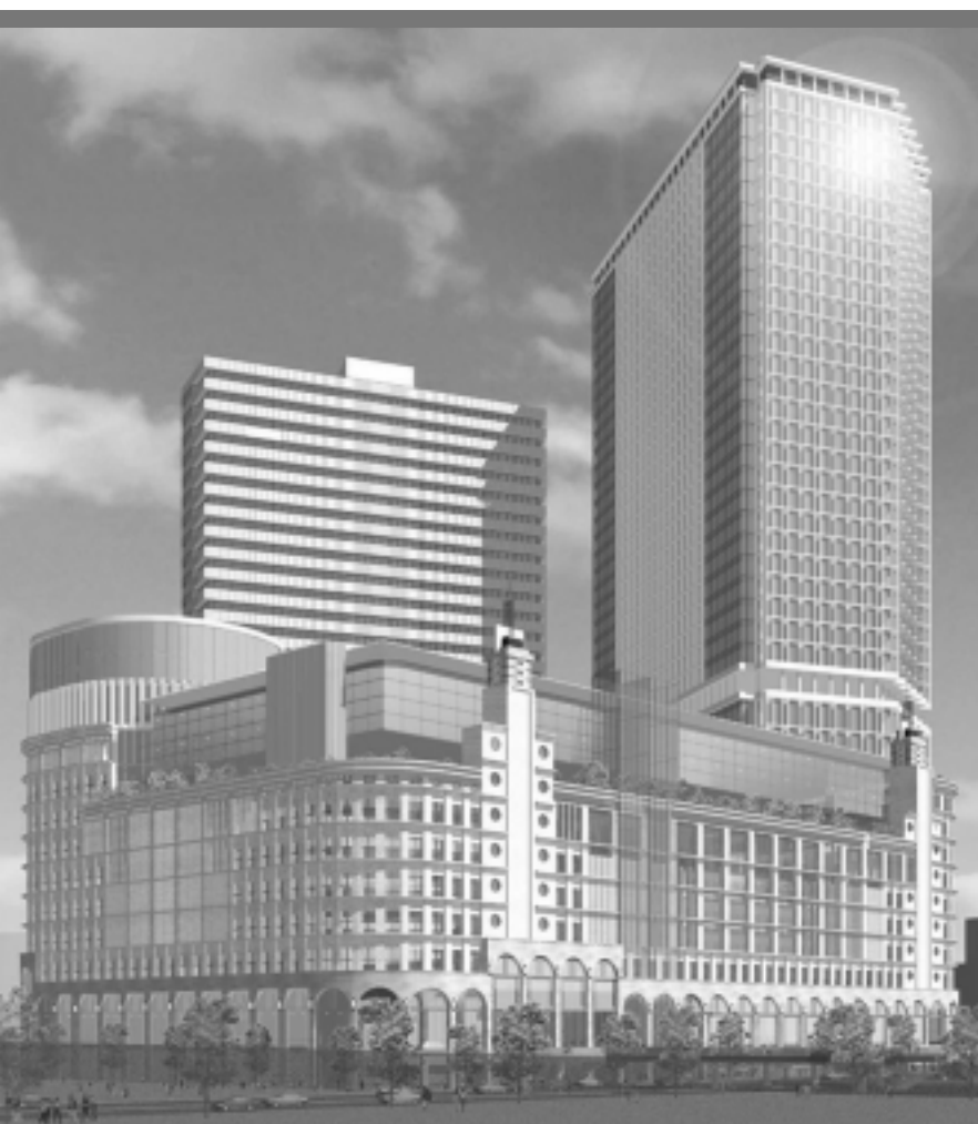
New Umeda headquarters externals image
