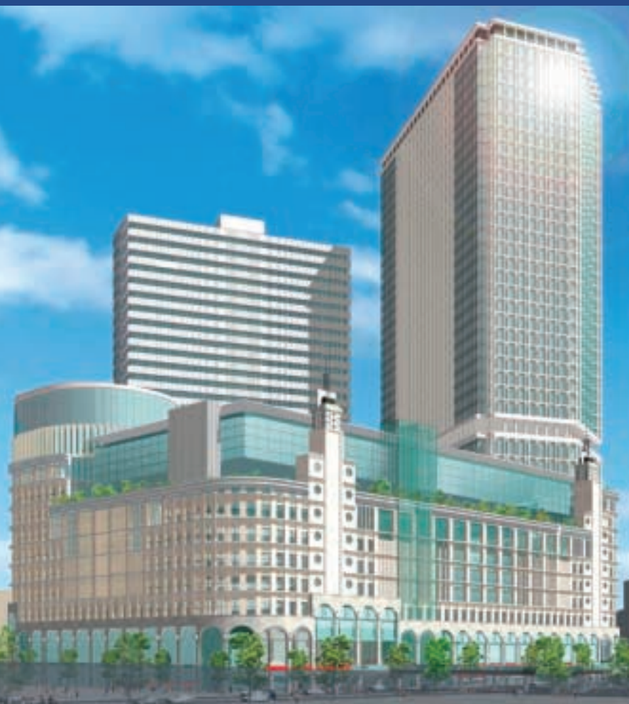
Exterior view of new Umeda Main Store
