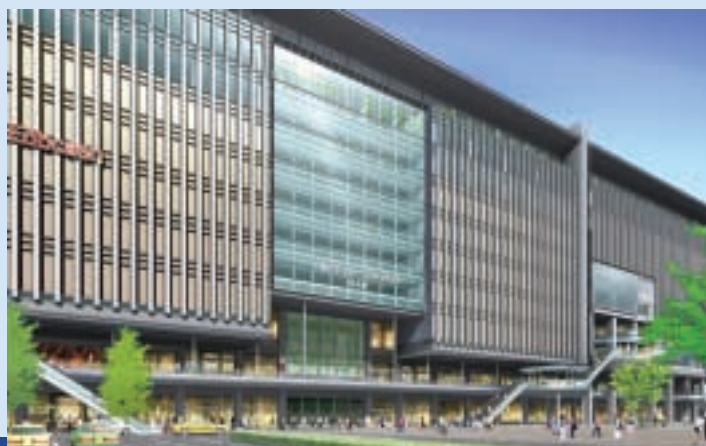
Exterior view of New Hakata Station Building
