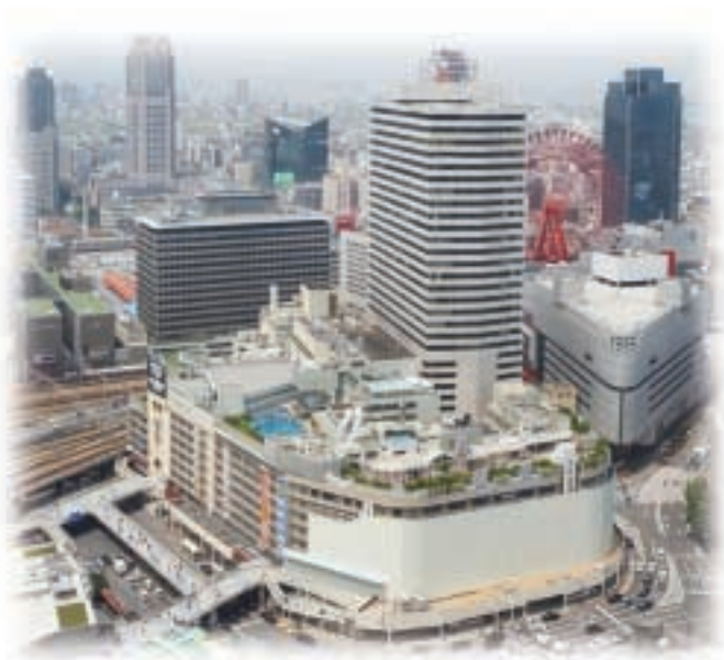
Umeda Main Store under construction
